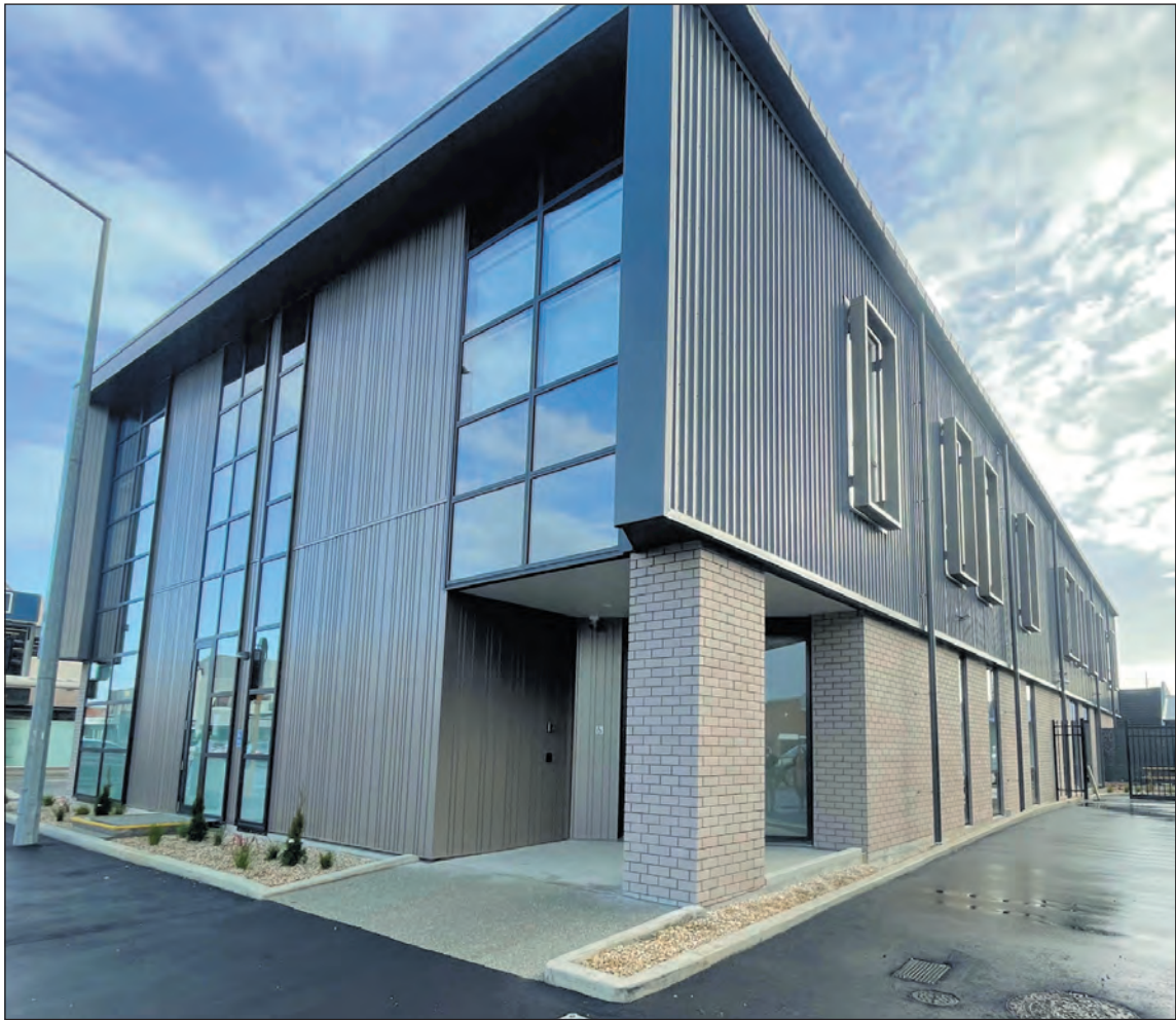
A long way south, but with Mid Canterbury firmly in mind. Somerset Ashburton Trust's new $8 million Invercargill commercial property is now open, with income from the DOC-tenanted building ultimately helping fund organisations, projects and people back in Mid Canterbury.
